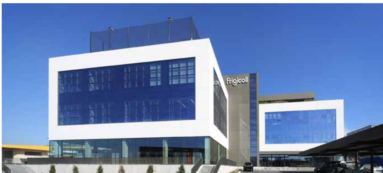
FRIGICOLL CENTRAL OFFICES
